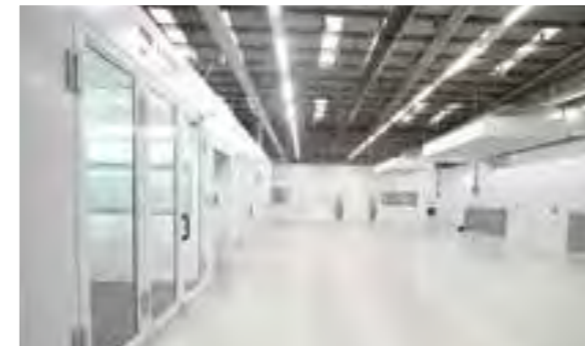
LIGHTING AND VENTILATION
