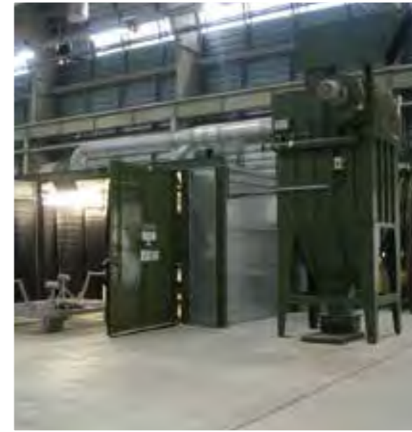
MANUAL BLAST FACILITY
