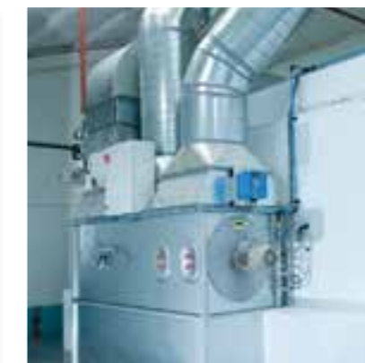
ENERGY-EFFICIENT AIR HANDLING PLANT
