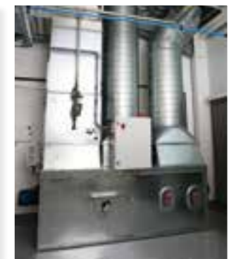
ENERGY-EFFICIENT AIR HANDLING PLANT
