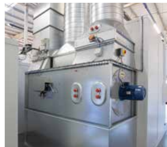
ENERGY-EFFICIENT AIR HANDLING PLANT
