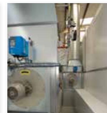
ENERGY-EFFICIENT AIR HANDLING PLANT
