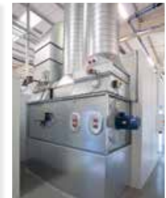
ENERGY-EFFICIENT AIR HANDLING PLANT
